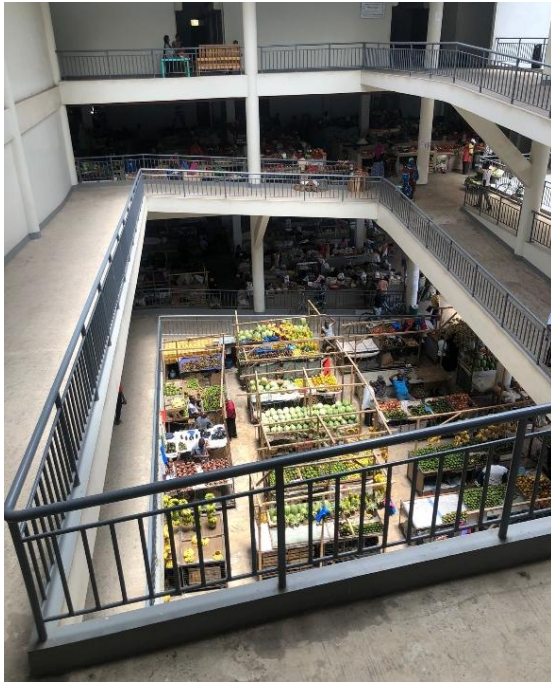
Atrium structure, Magomeni, 2022
