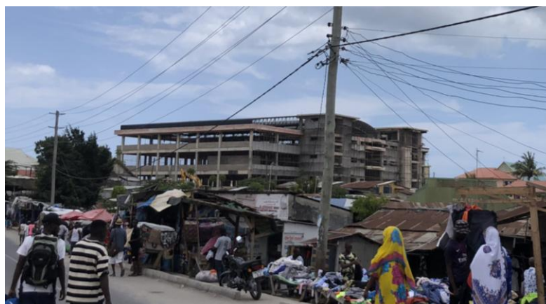
Houses and shops around Tandale (under construction)
